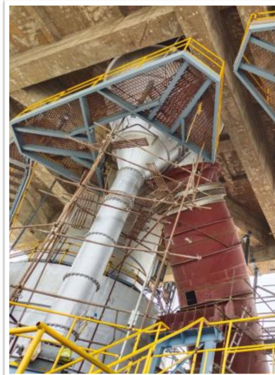
CCX cyclone installed at preheater top cyclone-Latest Technology by FLS
