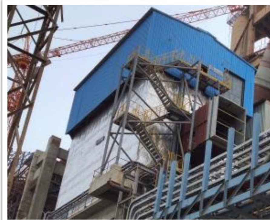
Kiln+RM bag house & Coal mill
