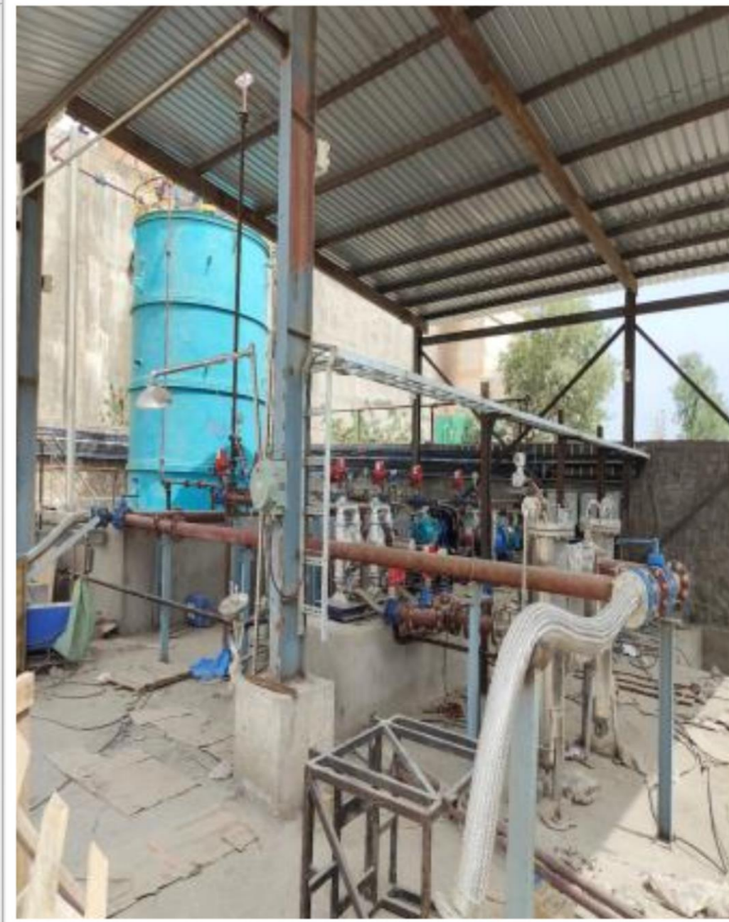
Fully automated PH1 Liquid AFR feeding system
